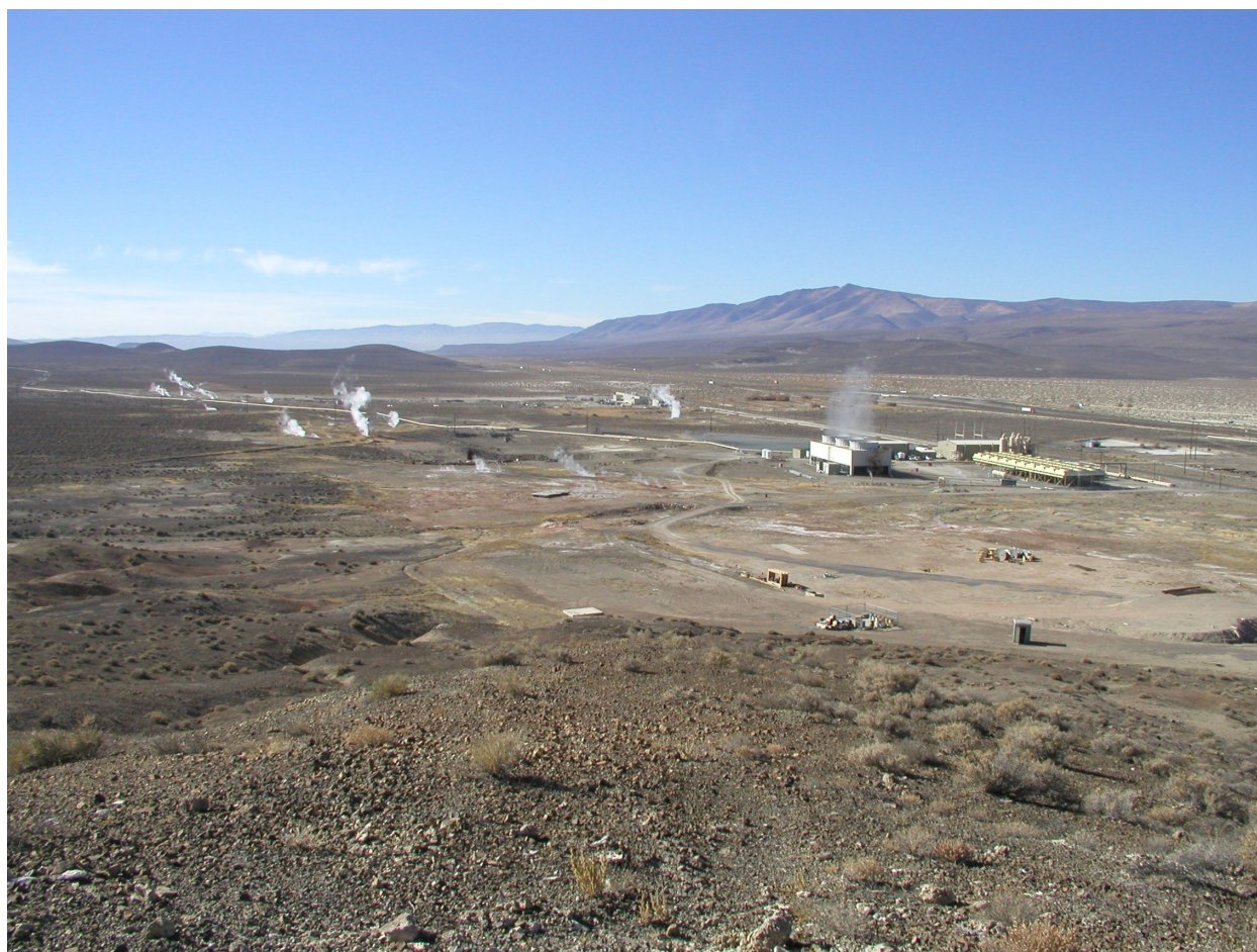
Figure 1. View of Bradys geothermal plant and steam vents with I-80 in the background (Photo by Mark Coolbaugh, November 2002).
